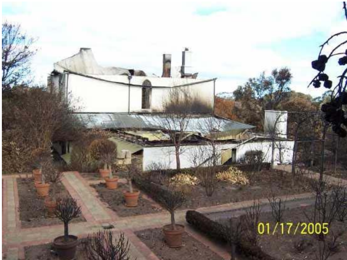
A destroyed heritage building in Green Patch, near Port Lincoln.
