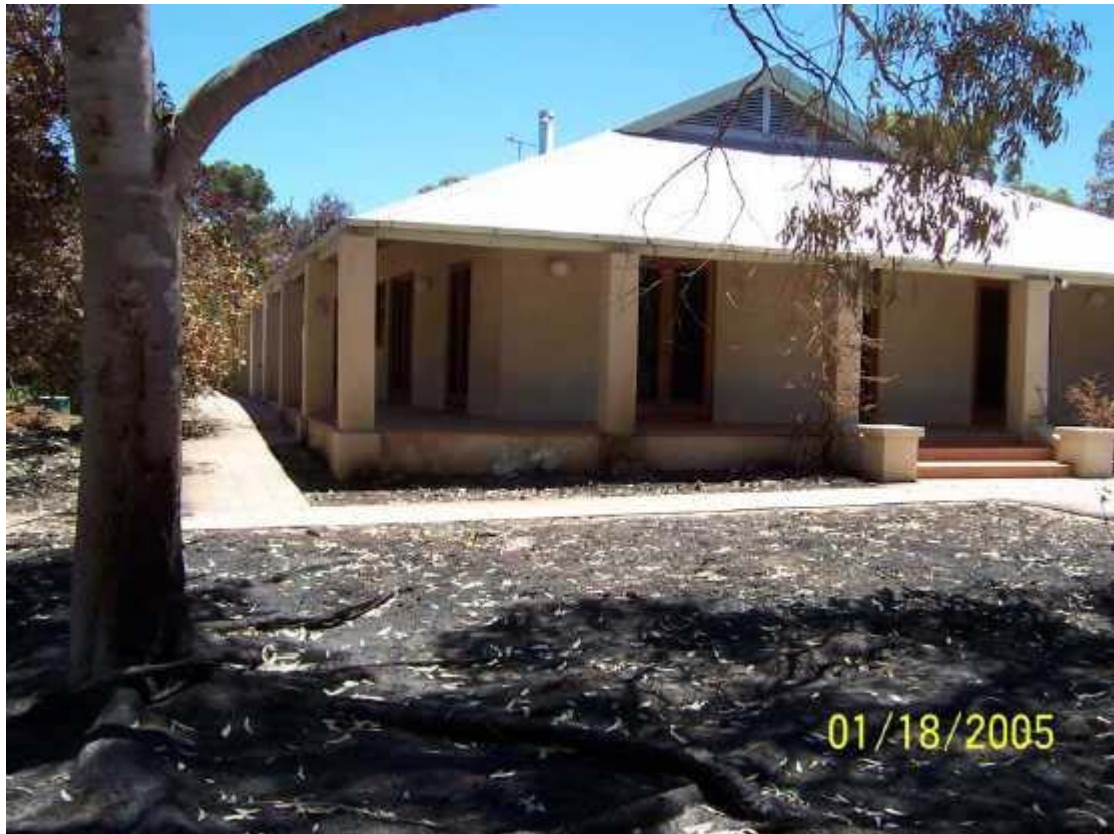
Property damaged in North Shields, near Port Lincoln.
