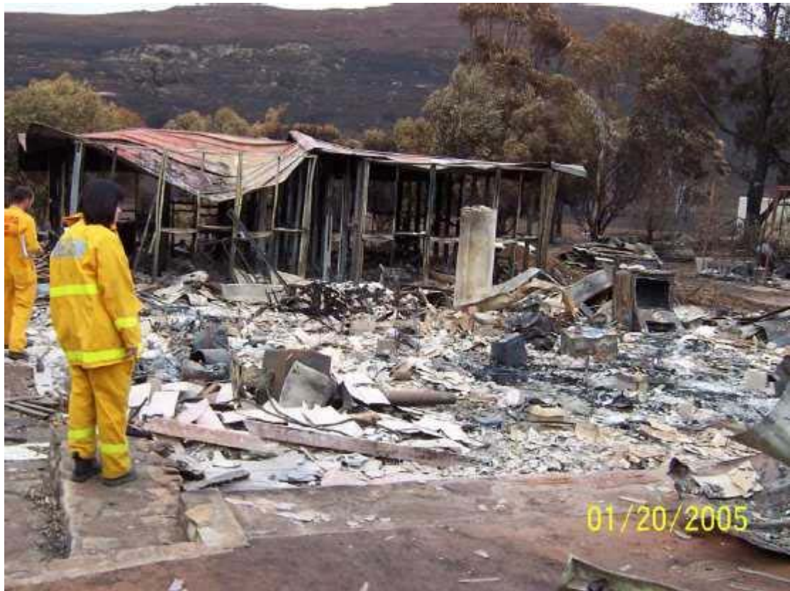
Personnel from the Country Fire Service (CFS) and CSIRO surveying the damage to a building destroyed in Whites Flat, near Port Lincoln.
