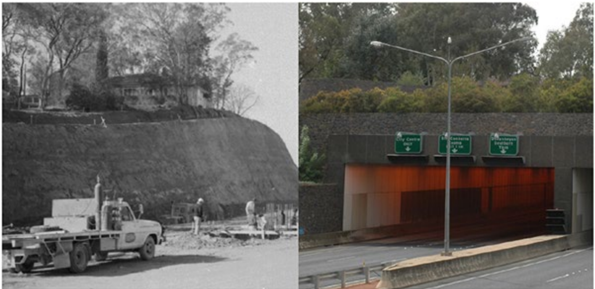
Figure 1: This pair of photos show the Molonglo Parkway (the west end of Parkes Way). The 1977 photo shows the cutting at ANU before it was covered to form the tunnel. At that time the then Bureau of Mineral Resources (now Geoscience Australia) carried out geotechnical studies for the alignment of the Molonglo Parkway from Acacia Inlet to Sullivans Creek.
