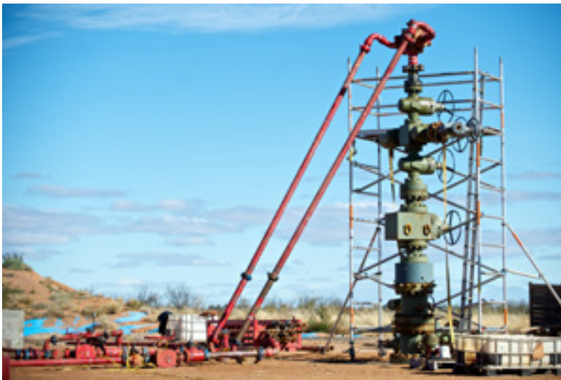
Figure 1: Hydraulic stimulation at the Paralana-2 wellhead. Courtesy of Brooke Whatnall (The Advertiser Newspaper) via Petratherm Ltd.
