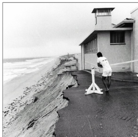
Plate 2.10: Coastal erosion on Perth's beaches (Courtesy of West Australian )
