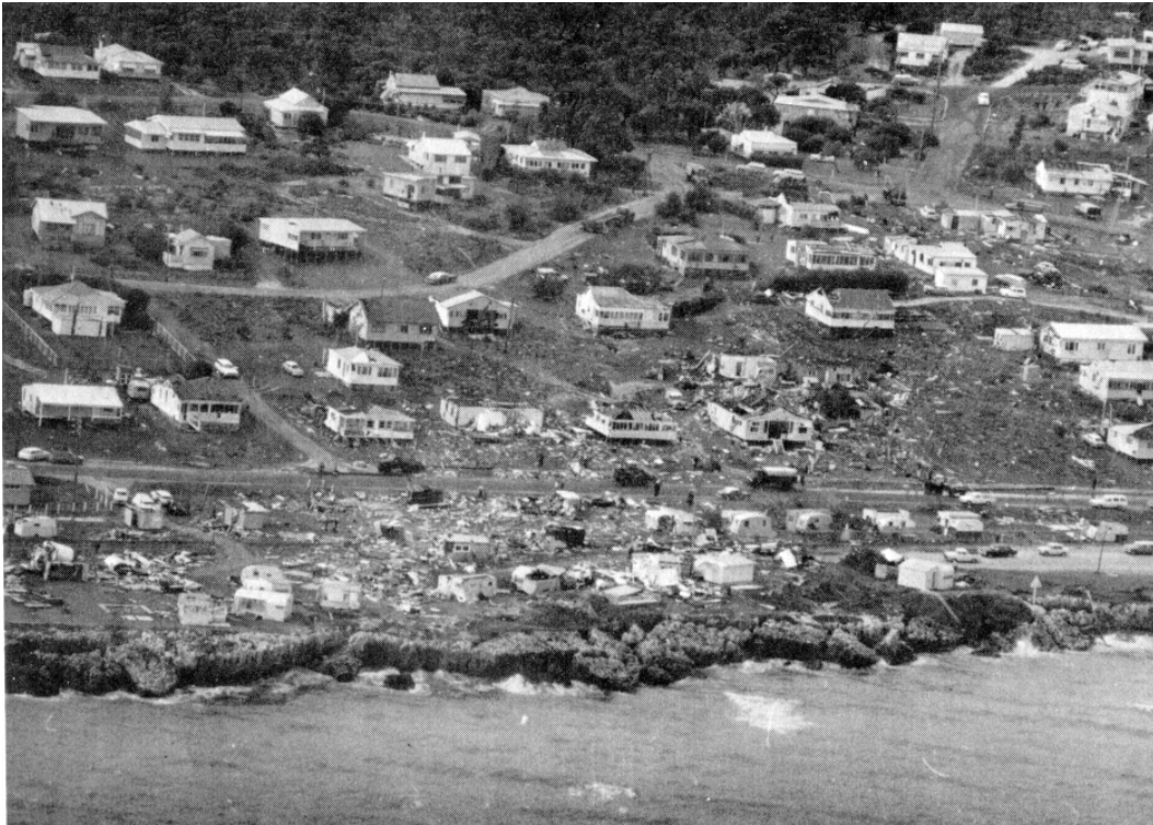
Plate 2.1: Damage from the tornado at Naval Base, 8 June 1968 (Courtesy of the West Australian )
