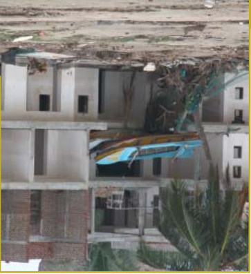
Figure 5: Two small boats stranded on the first floor of a building after the 2004 Indian Ocean Tsunami. (Nalini Kasynathan – courtesy OxfamCAA)
