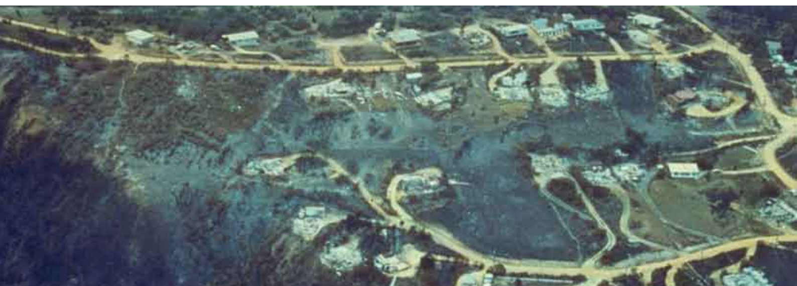
Aerial view of the devastation caused by the Ash Wednesday fires at Fairhaven, Aireys Inlet, Victoria, February 1983 Photo courtesy: Emergency Management Australia.
