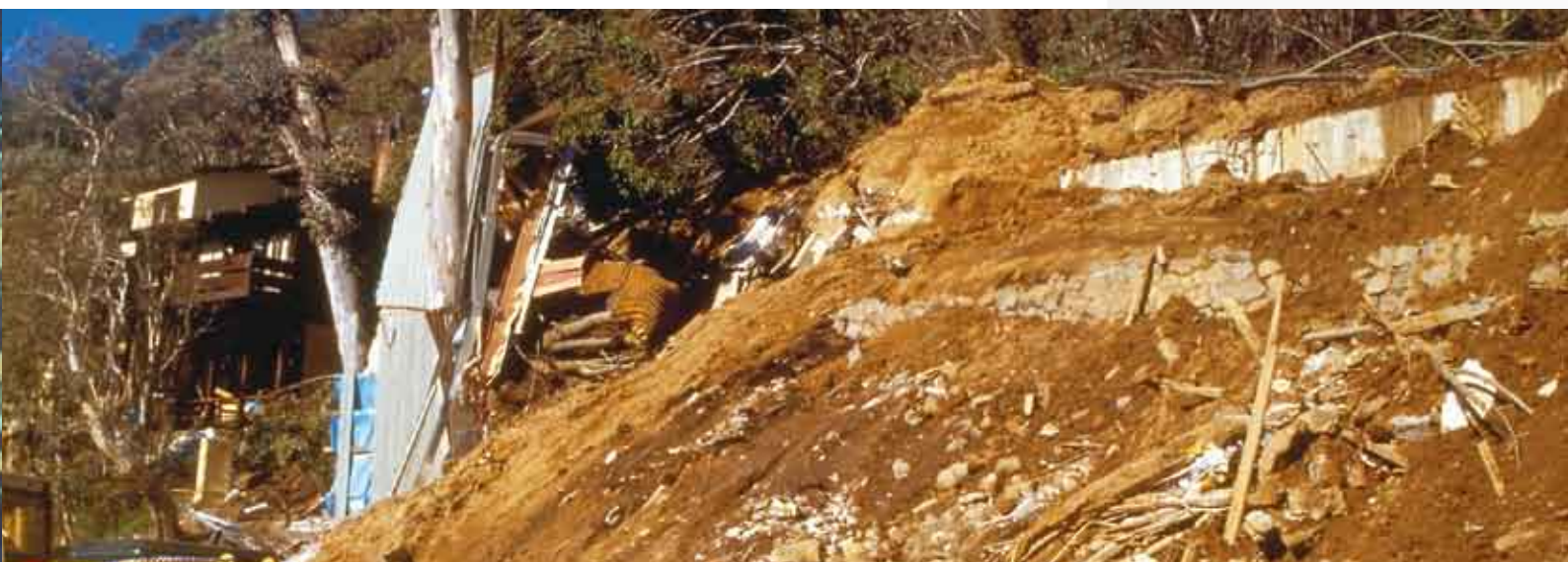
Side view of a fatal landslide at Thredbo, New South Wales, July 1997 Photo courtesy: Geoscience Australia.
