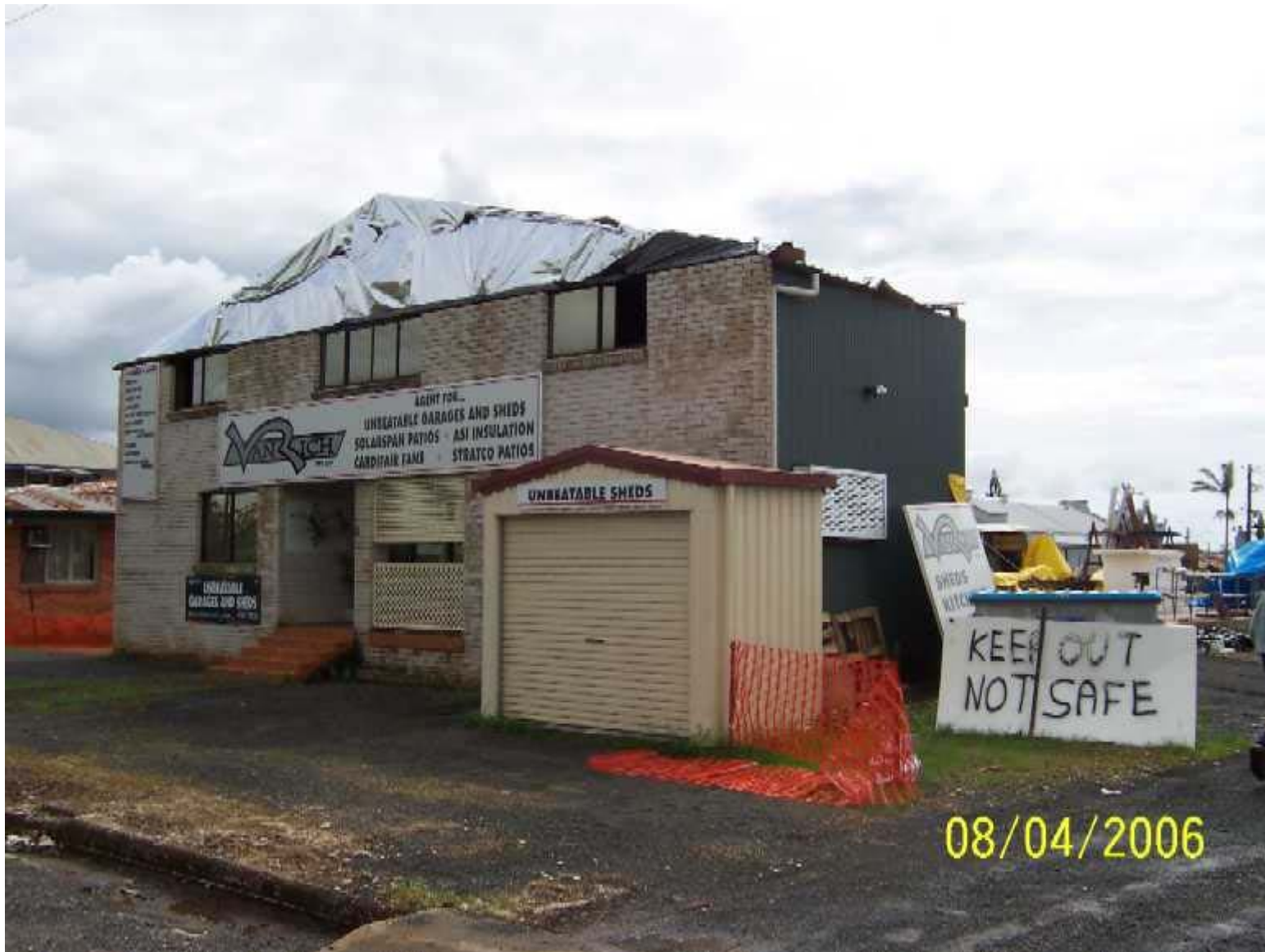
Destroyed industrial building following Cyclone Larry, Innisfail. Image courtesy Geoscience Australia.
