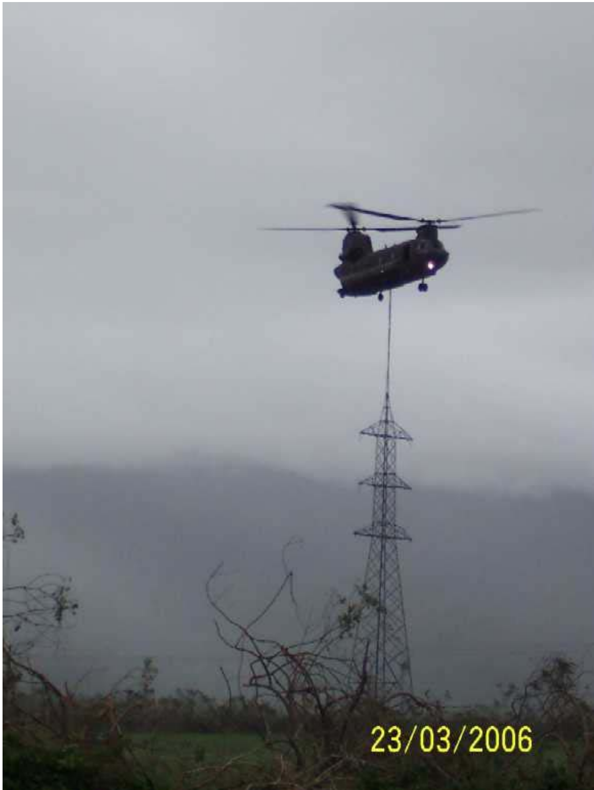
Helicopter replacing and restoring power to Innisfail. Image courtesy Geoscience Australia.
