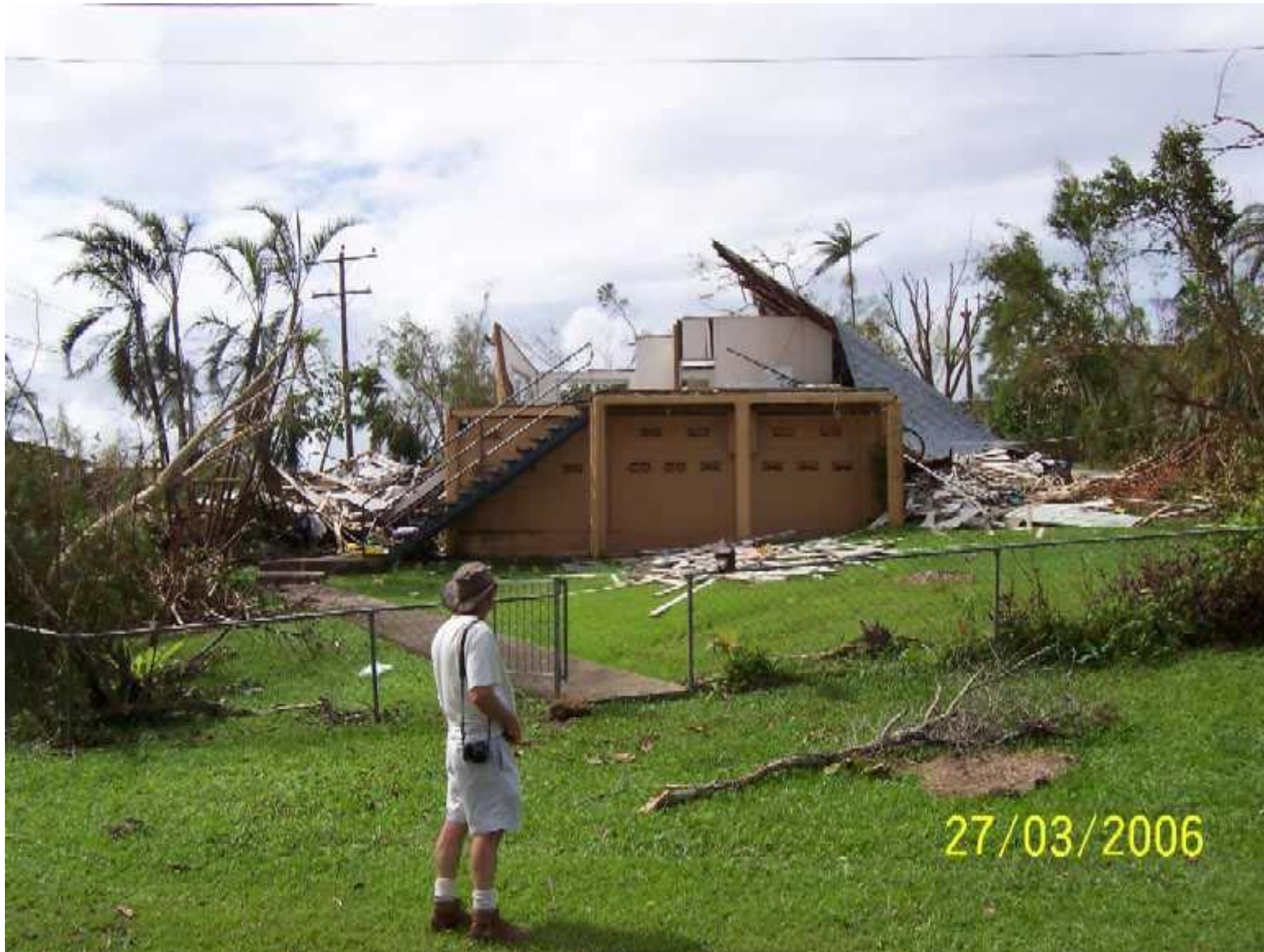
Destroyed residential building following Cyclone Larry, Innisfail. Image courtesy Geoscience Australia.
