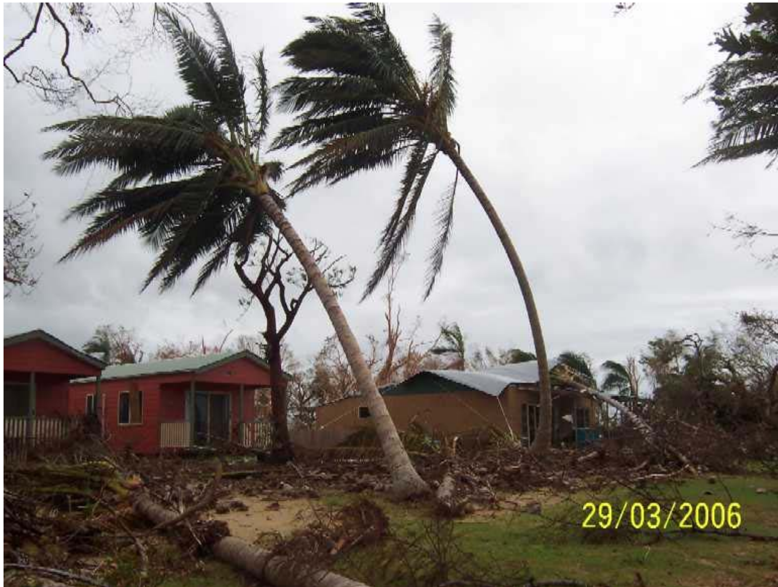
Tree damage to residential buildings following Cyclone Larry, Innisfail. Image courtesy Geoscience Australia.
