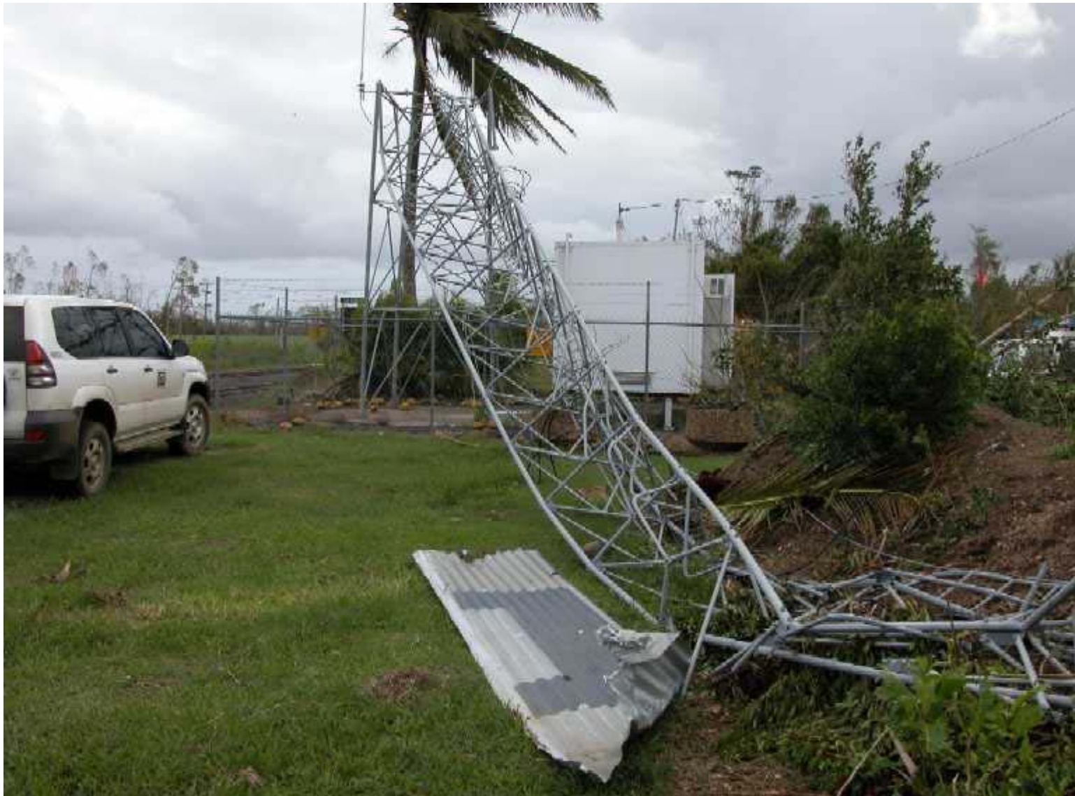
Antenna damaged by Cyclone Larry, Innisfail. Image courtesy Geoscience Australia.
