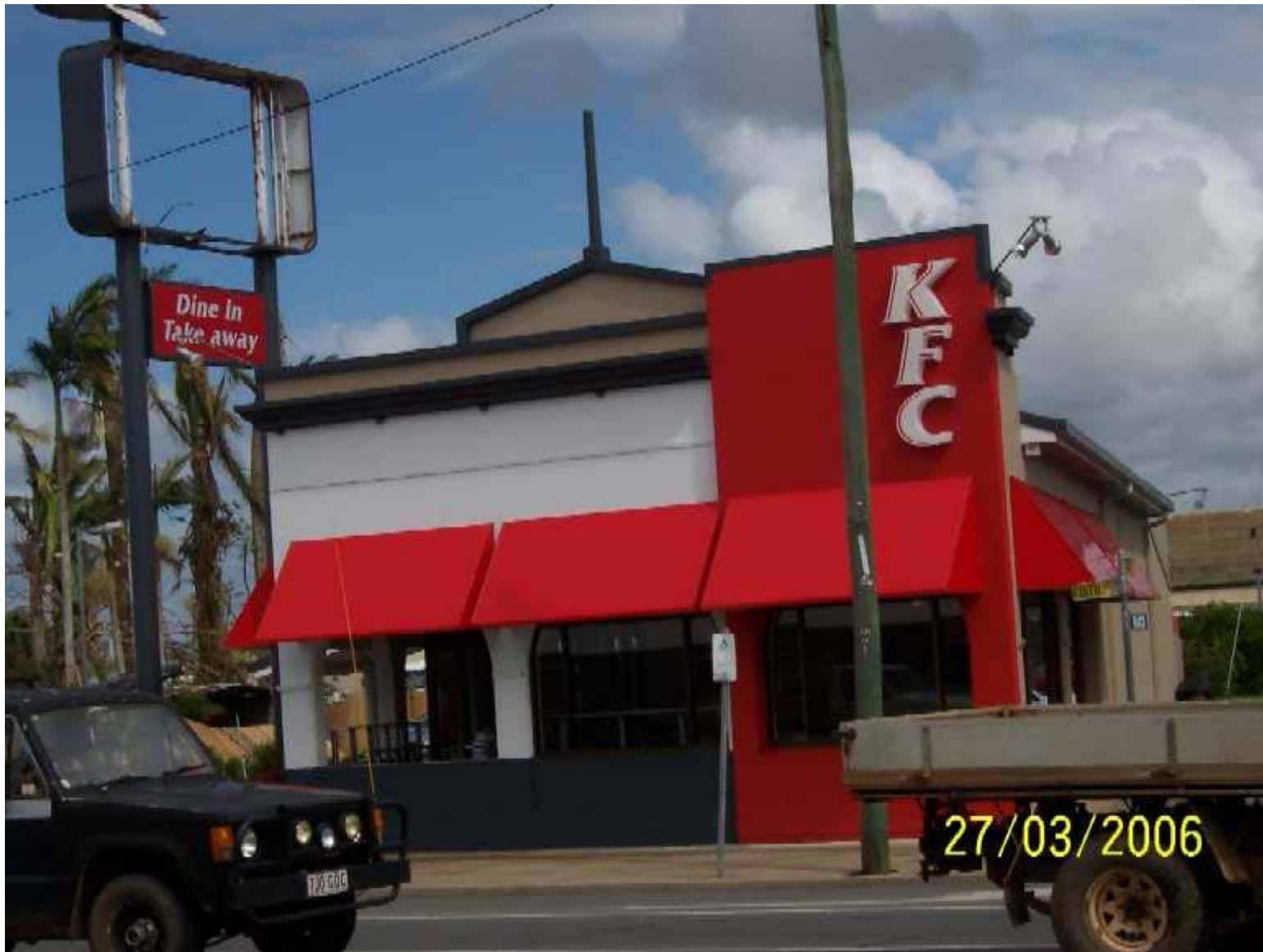
Commercial building damage following Cyclone Larry to "KFC", Innisfail. Image courtesy Geoscience Australia.
