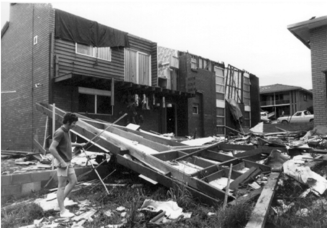
Figure 6. 10 Tornado damage from the November 1973 event in Brisbane
