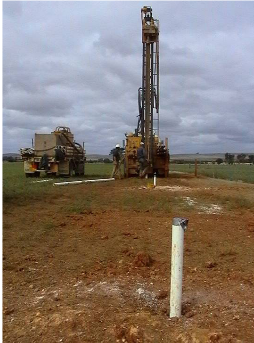
Figure 4: Nested piezometer construction
