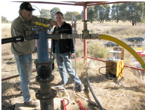
Figure 20: Install diversion T-piece between bore headworks and outlet
