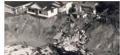
Figure 2. Coastal erosion at Wamberal beach, New South Wales, in 1978.
