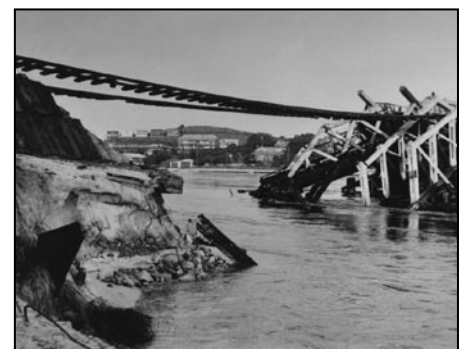
▲ Figure 3. Fremantle Railway Bridge destroyed by the July 1926 floods (photo courtesy of The Batty Library 54902P).
