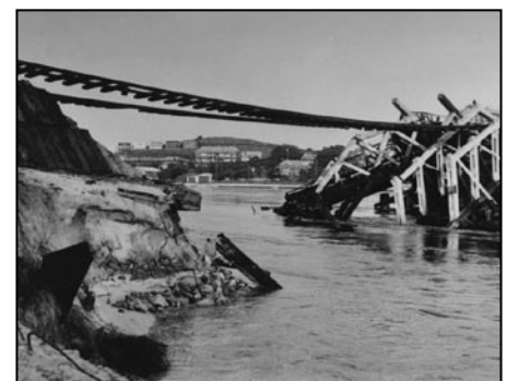
▲ Figure 3. Fremantle Railway Bridge destroyed by the July 1926 floods (photo courtesy of The Battye Library 54902P).
