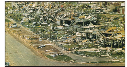
▲ Figure 1. Housing estate destroyed by Cyclone Tracy in 1974 (Bureau of Meteorology).
