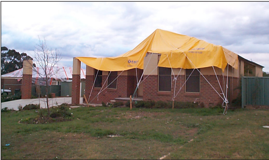
◀ Figure 2. Housing damaged by a tornado in Bendigo, Victoria, in May 2003 (Geoscience Australia).
