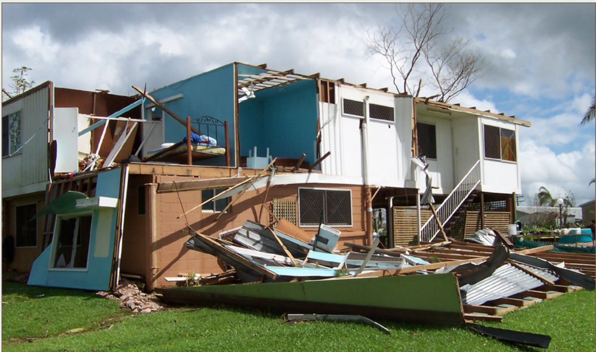
Figure 1. Damage to pre-1980s dwelling in Innisfail from Tropical Cyclone Larry.
