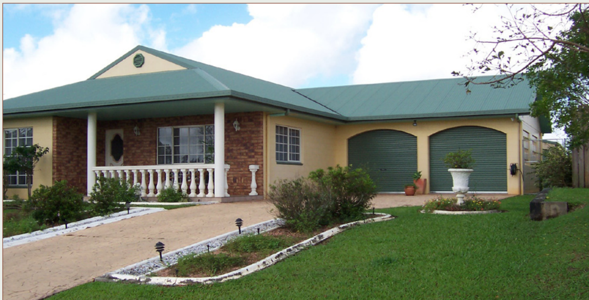
Figure 2. Dwellings constructed after amendments to the Queensland Building Act in 1981 withstood Cyclone Larry better. A systematic approach to assessing cyclone risk in other tropical Australian cities will reveal the relative risk from cyclones in each city and areas of higher risk within each city.
